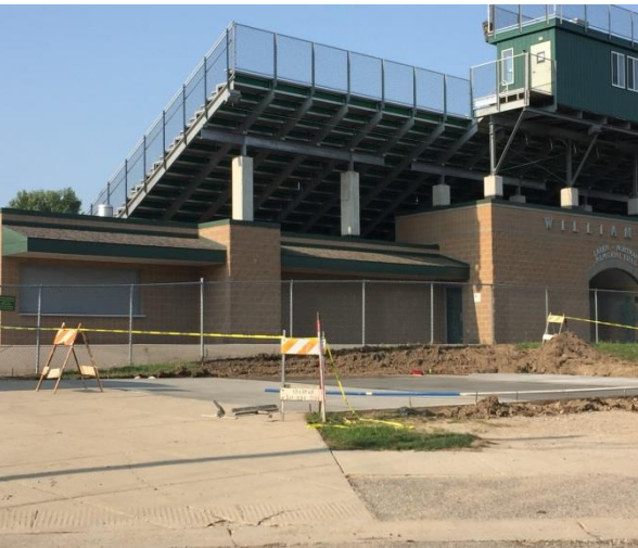
Sidewalk and Parking Lot Repair (Various locations) $25,000
