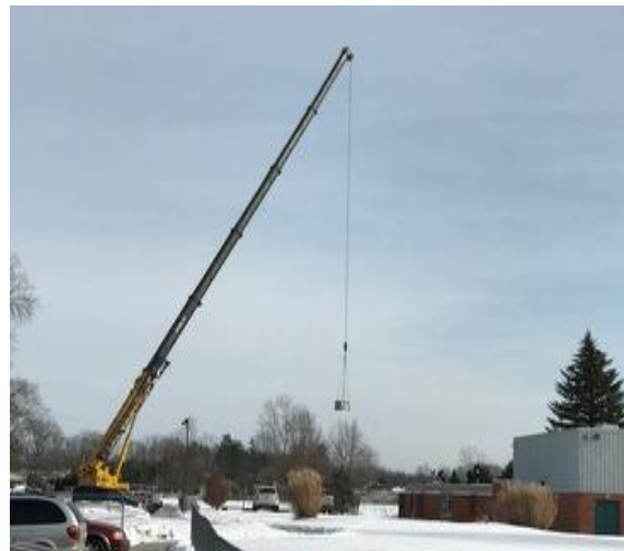
Rooftop Heating Unit Repair at Explorer Elementary and WHS $40,000
